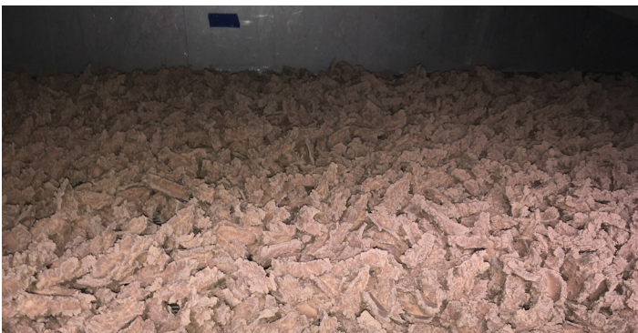
View into the second dryer module with granulated dry material
