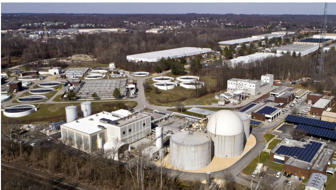
Little Patuxent Water Reclamation Plant (LPWRP)
