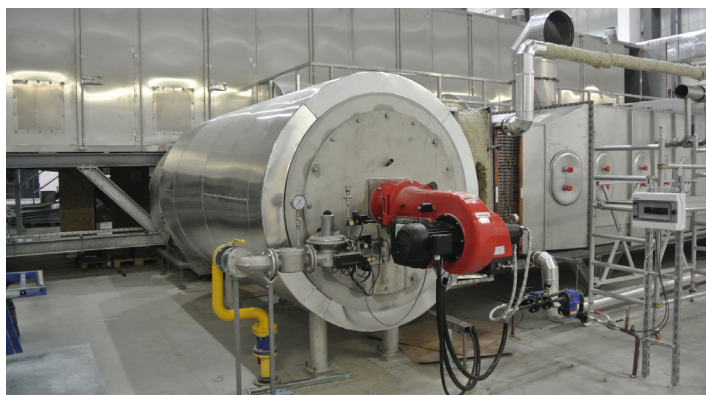
Burner plenum for natural gas with combustion chamber and blower for combustion air
