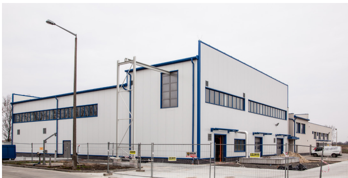
Exterior view building sludge treatment
