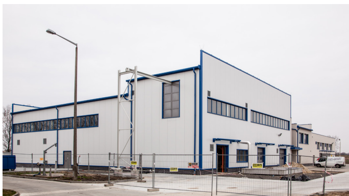
Exterior view building sludge treatment
