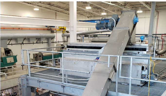
Chain conveyor (wet product) to inlet unit (Distributor-/Dosing-unit)
