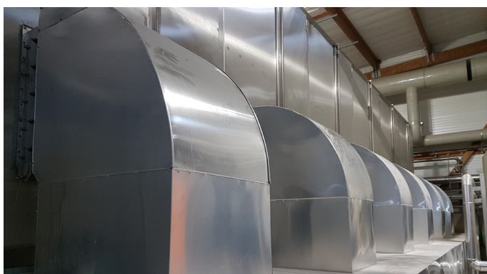
Belt dryer BD 3000/7 with exhaust air ducts
