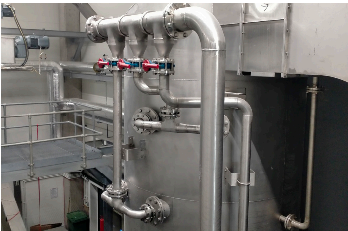
Preheating of the digested sludge in countercurrent column with humid warm exhaust air of the Belt Dryer
