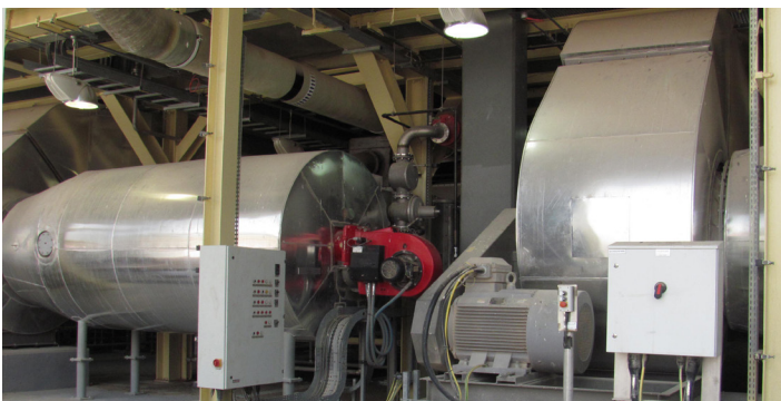
Burner (red) with combustion chamber and supply air fan
