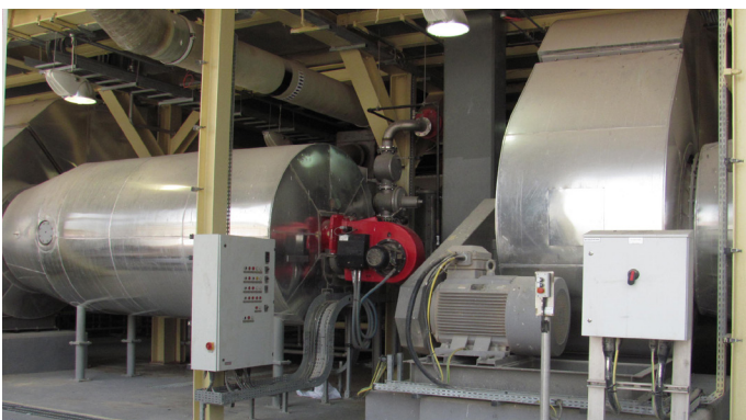
Burner (red) with combustion chamber and supply air fan
