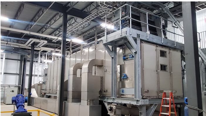
Belt Dryer BD 3000/6 with feeding unit, discharge screw, inlet air duct
